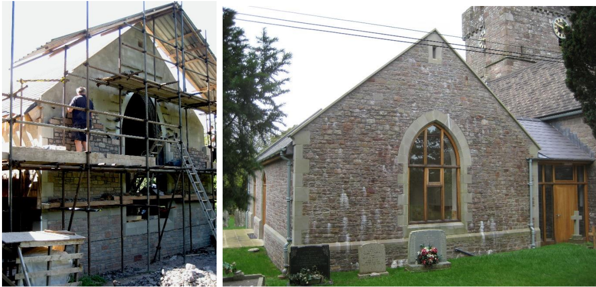
The partly constructed building covered in scaffolding and the finished extension
