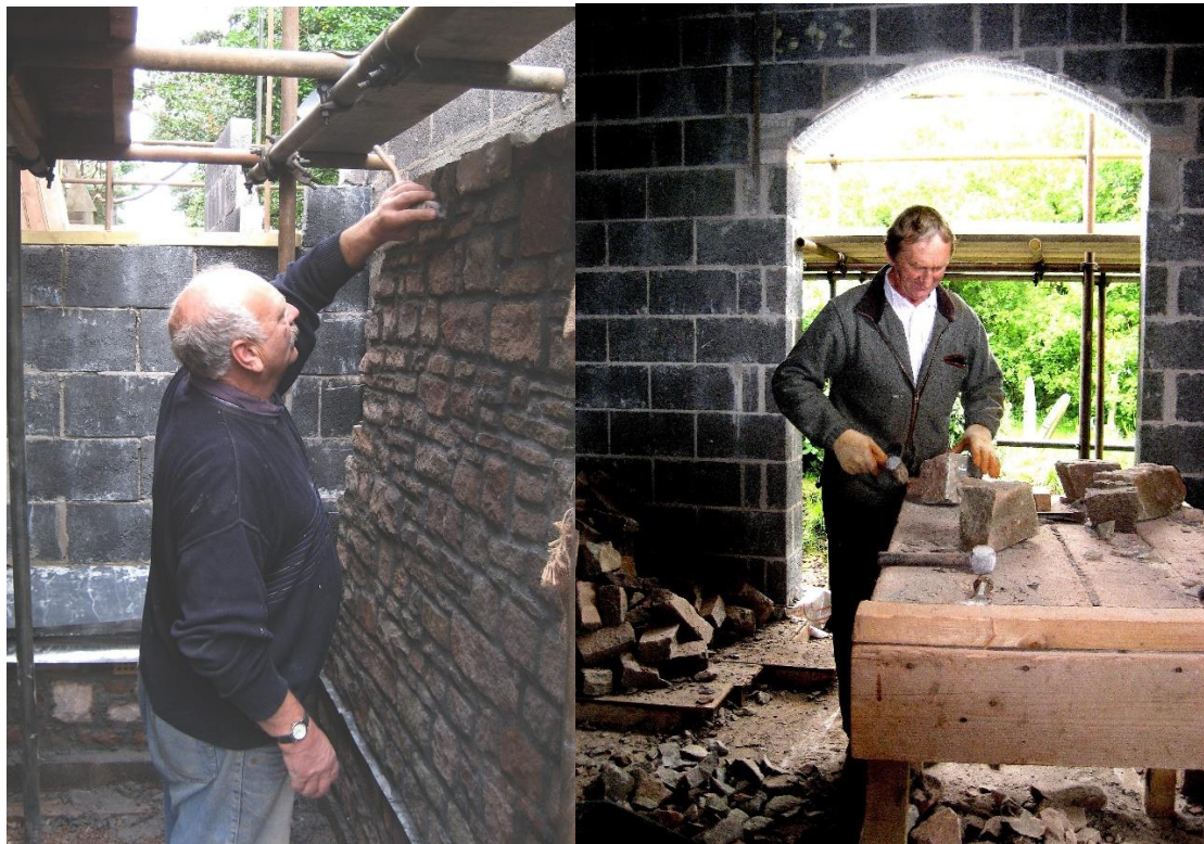
John Saysell pointing the stonework and a stone cutter making sure the angles are right
